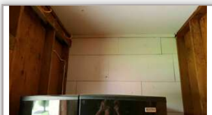
CARPORT SHED INTERIOR WALL
