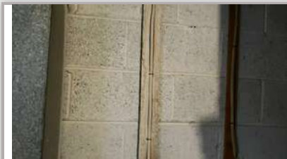
CONCRETE BLOCK FOUNDATION
