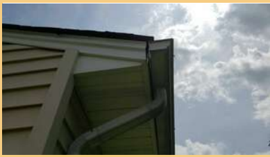
REAR AT CARPORT
