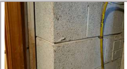
CONCRETE BLOCK FOUNDATION
